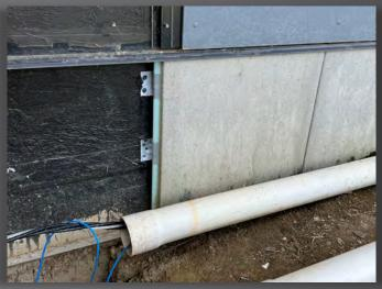
WallGUARD® panels are installed using specially designed galvanized steel mounting clips, which are
