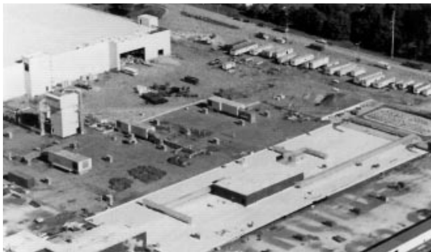
A T. Clear Protected Membrane Roof System, using LIGHTGUARD Protected Membrane Roof Insulation, protects the membrane from damage by heavy construction traffic during plant renovations.
