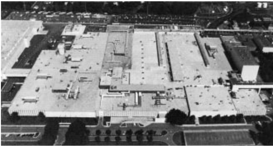
Once installed, a T. Clear Protected Membrane Roof System, using Lightguard PMRI, offers a lightweight, yet durable alternative to conventional ballasted systems.
