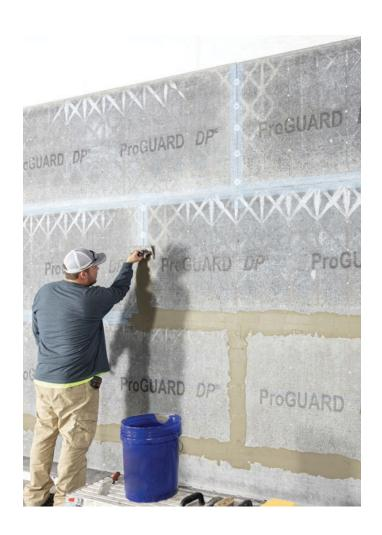
ProGUARD *DP*® consists of a nominal 1/4" thick Util-A-Crete® concrete backerboard that is reinforced with two layers of fiberglass mesh. The Util-A-Crete® fiberglass reinforced concrete surface of ProGUARD *DP*® has a compressive strength of 2600 psi providing a hard durable surface that is resistant to impact. This concrete panel is laminated to extruded polystyrene, expanded polystyrene or mineral wool insulation in standard thicknesses.
