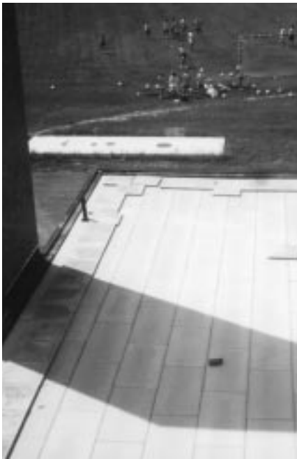
Top Left: A brick thrown or fallen from a nearby chimney does no damage to this LIGHTGUARD Protected Membrane Roof at Chateaugay School.
