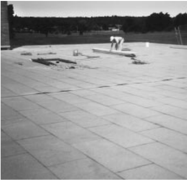
Above: A workman walks on this LIGHTGUARD Protected Membrane Roof while doing repairs to the chimney at left.
