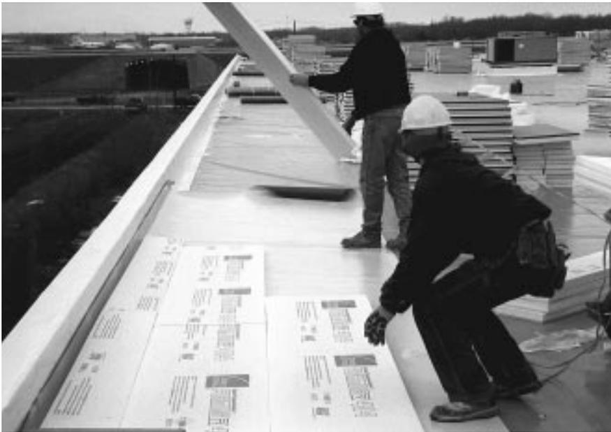
Workers from Progressive Roofing, Inc. are exposed to the wind and cold as they install this Heavyguard Protected Membrane Roof System.
