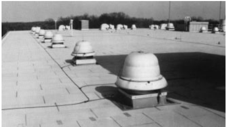
LIGHTGUARD provides flexibility in handling roof features such as blowers and vents.
