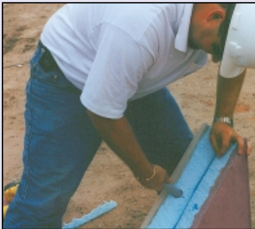
Contractor installs custom designed fasteners to Lightguard panel.
